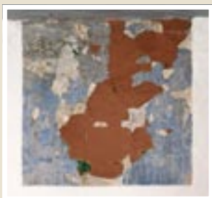
Paint traces on wall, east entrance.
