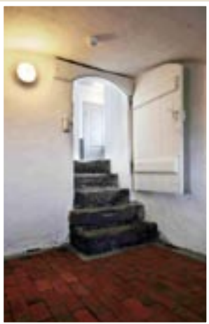
Original cellar stairs.
