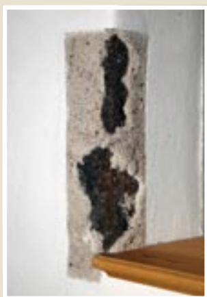
Icelandic basalt with Danish lime mortar in window surround, upper floor.
