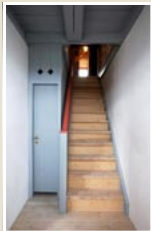
Remade staircase, east entrance.
